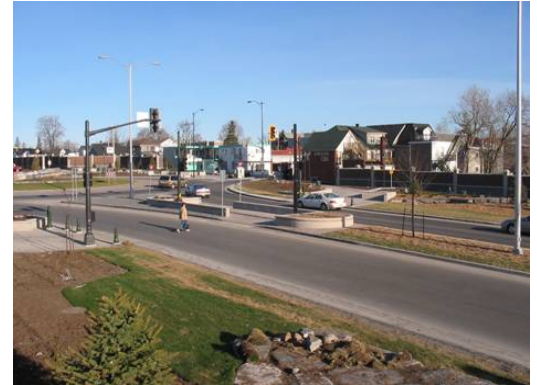
Figure 3. Example of Off-Set or Staggered Crosswalk Condition
